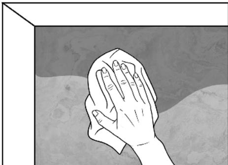
Dampen a dry cloth with Akemi water repellent product and protect the stone evenly. The water repellent will remove excess glue at the same time (within 10 minutes after installation). 20 minutes later : remove the excess product with a clean cloth.
